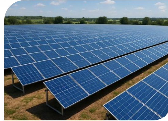
France: Agrivoltaic power plant for Reden Solar in Montréal
