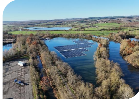
France: Geugnon floating PV project
